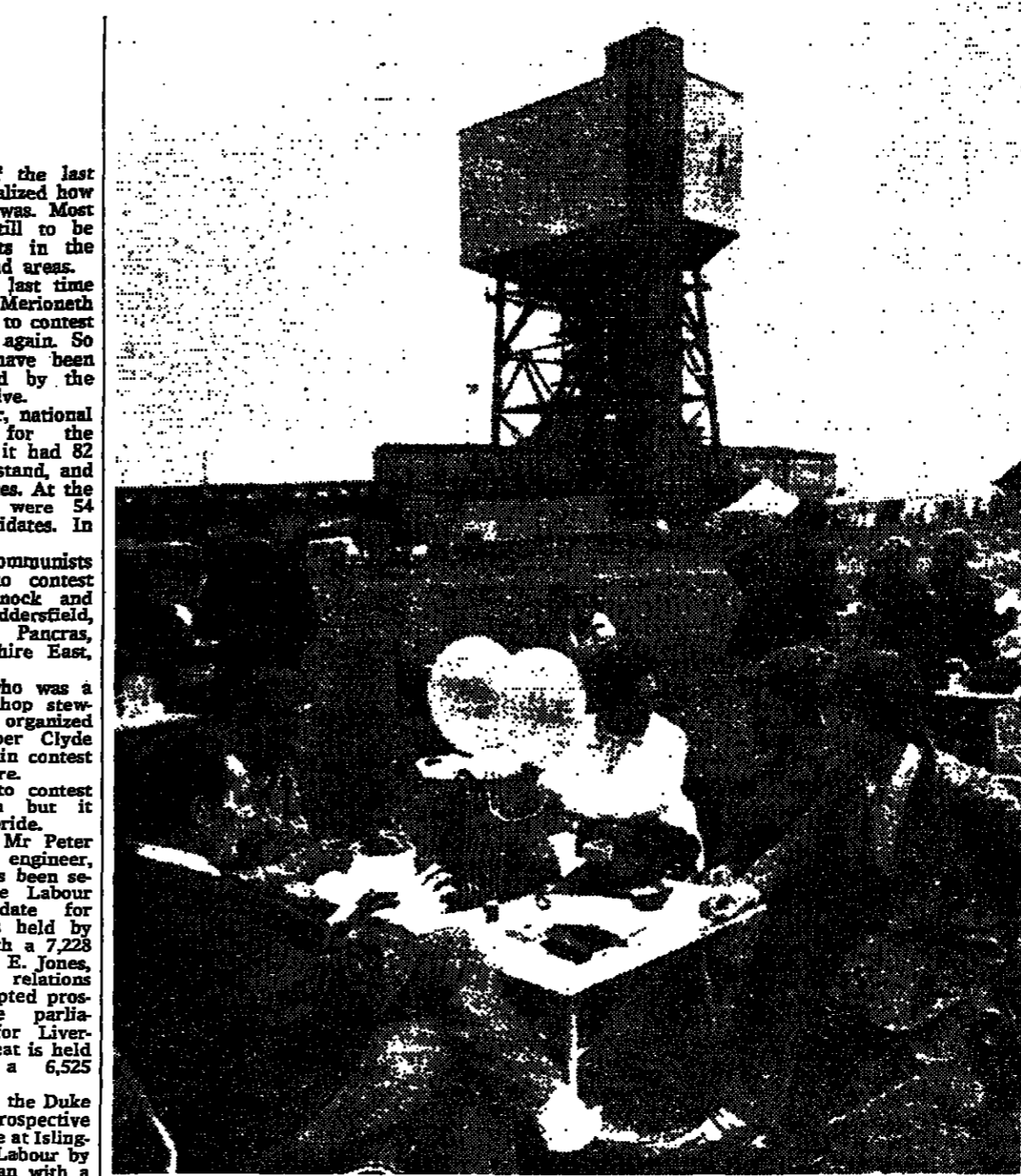
Picnic tea on the surface at Kellingley colliery open day yesterday.
